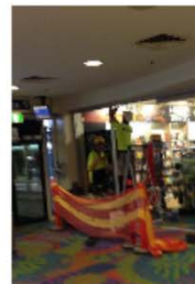
Unacceptable – inadequate barrier
