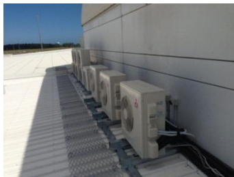
Photo 7.4.1 - shows walkway in Area A at west end.
